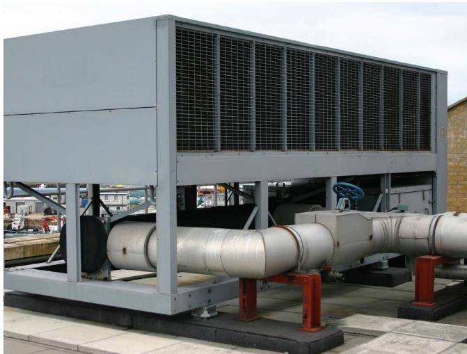
The basic principle behind the operation of a chiller is similar to conventional air conditioning in that the cooling is provided by refrigerant evaporation. However, there are significant differences, including the fact that chillers typically use water as the primary cooling medium rather than air. Chillers are generally large systems, often found in medium to large commercial and industrial facilities.
