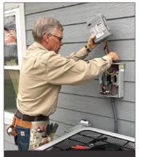
Energy Services Electrician Milt replacing a load control device
