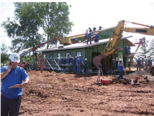
ECE crews working at the site.
